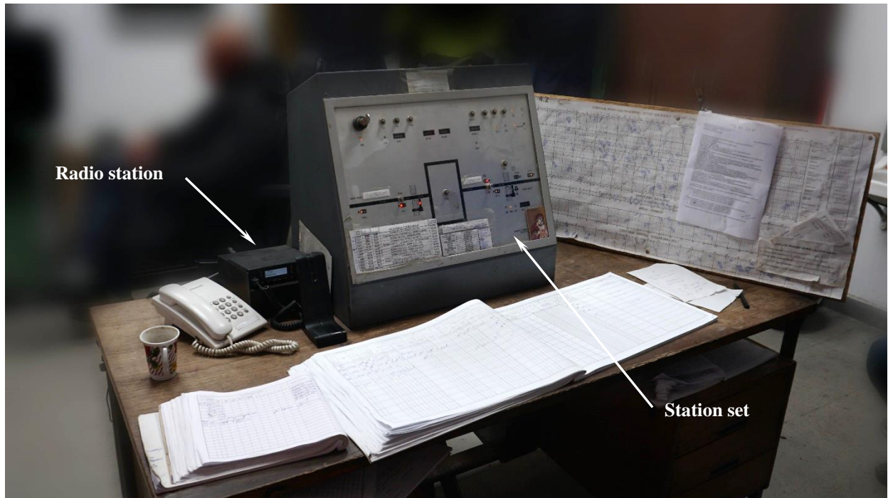
Figure 3.4.3.1: The appearance of the radio station and station set at the office of the train dispatcher of station Ratkovo
