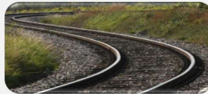
Track gage : 1435 and/or 1668mm Rail Inclination : 1/20 and/or , 1/30 and/or and/or 1/40
