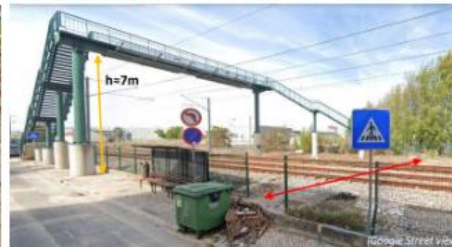
Illegal path B and designated footbridge
