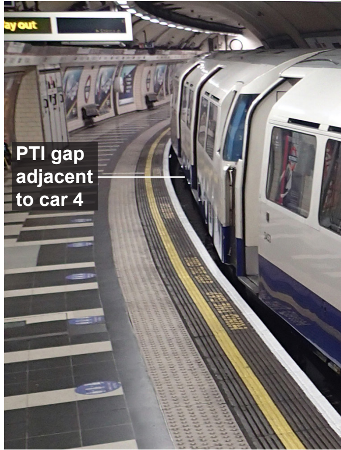
Figure 6: Platform-train interface gap adjacent to carriage 4 at Waterloo Bakerloo line platform 3
