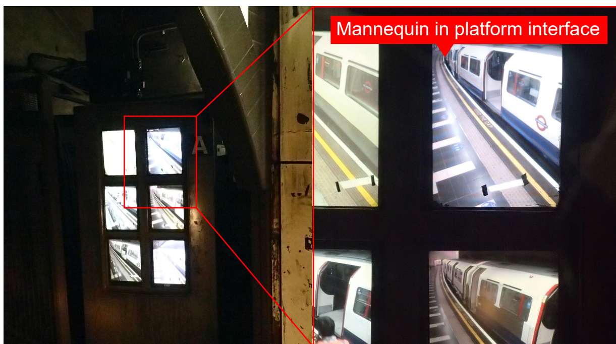
Figure 9: Layout of OPO monitors and position of passenger during despatch adopted by mannequin as would have been presented to operator of train 210 (inset)
