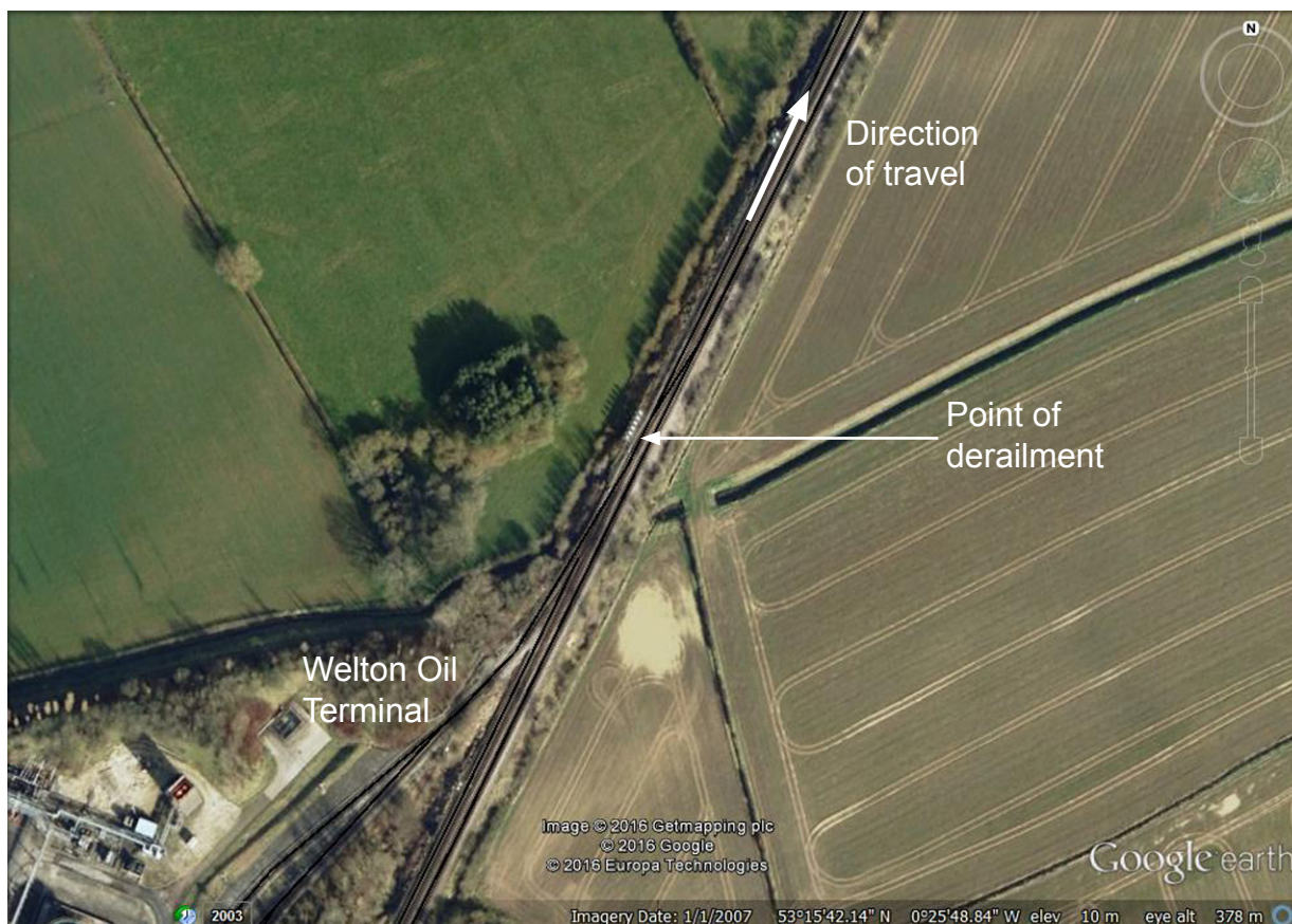
Figure 3: Google earth image showing location of derailment
