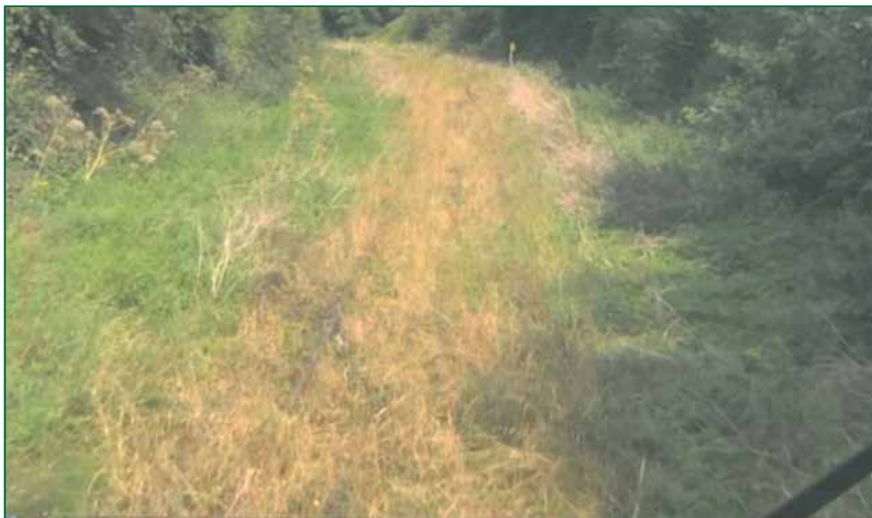
Figure 14: A section of the Antrim branch line with excessive weeds and lack of visibility of the track, September 2012
