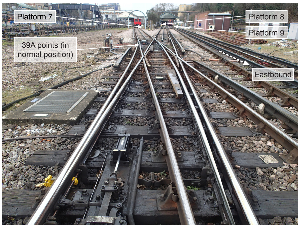
Figure 4: Showing the track layout from the east end of 38 points looking towards Ealing Broadway station. The train to the left is at platform 7 and the one to the right is at platform 9.
