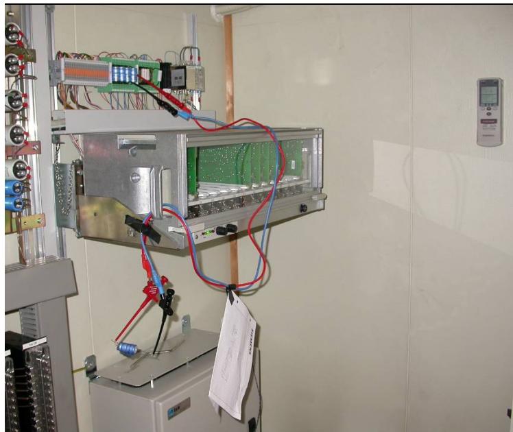
Figure 9: Interface system EF 180 at Slependen block signal station. This transmits signal information between the relay system at the block signal station and the computer-controlled interlocking system at Sandvika station via a telecommunications cable.
