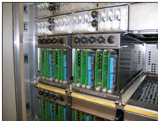
Figure 10: Picture of object controller for signal N 4323
