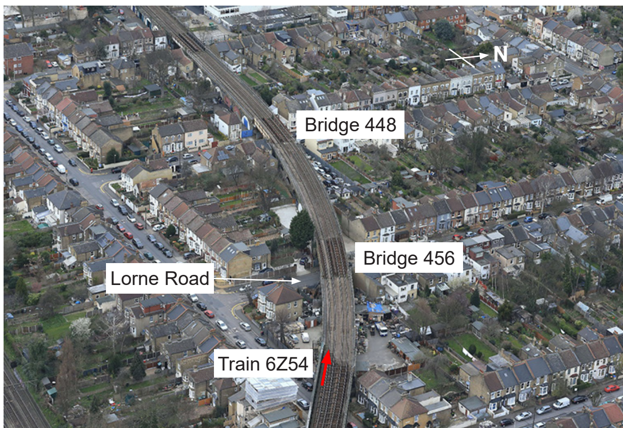
Figure 3: Aerial view of bridge 456 and bridge 448 looking north-west (courtesy of Network Rail)
