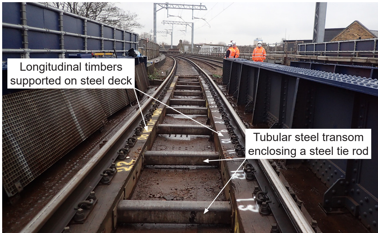
Figure 6: Bridge 456 up deck after removal of the deck walkway
