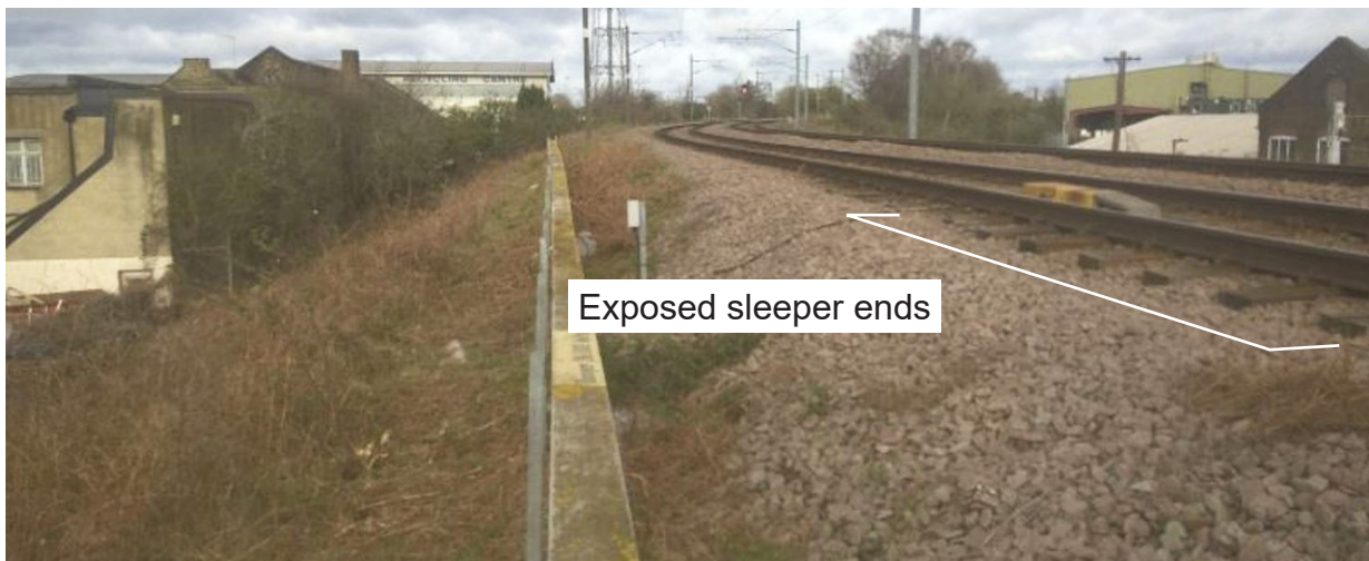
Figure 12: The condition of the up-side cess and ballast around 0 miles 27 chains on the up High Level lines as photographed during the specialists' site visit of 15 March 2019 (photograph courtesy SNC-Lavalin)
