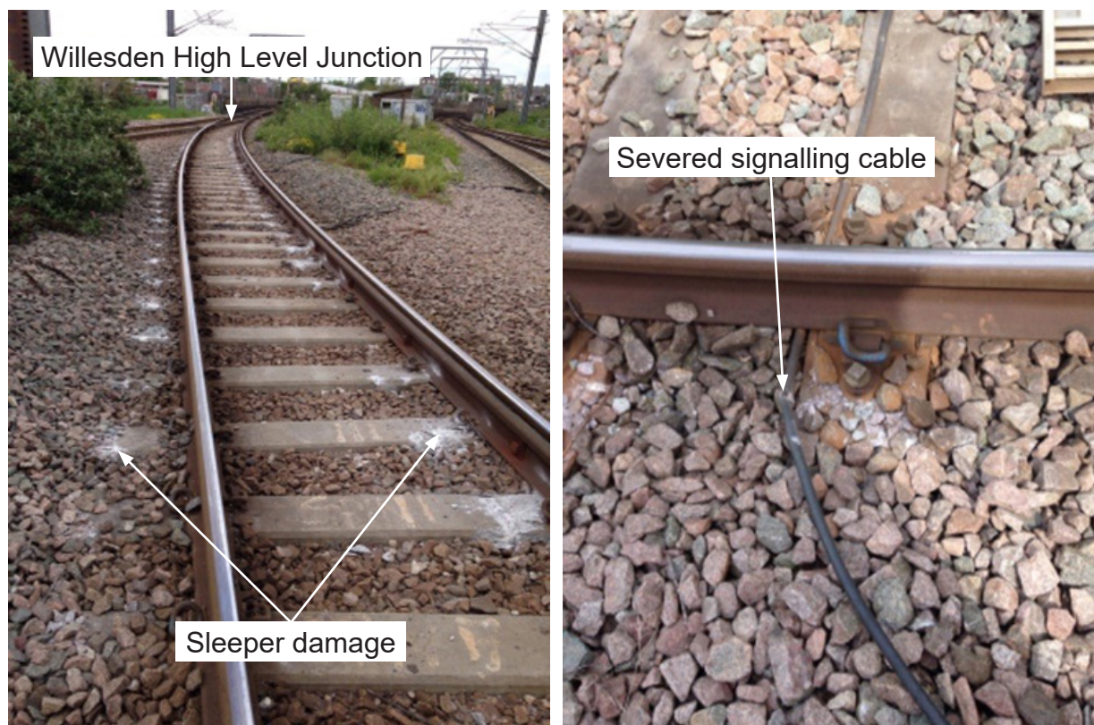
Figure 3: Reported track damage (photographs courtesy of Network Rail)
