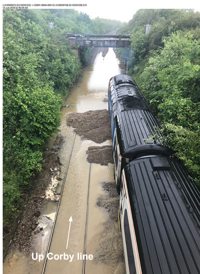
Figure 24: Flood water and sandy gravel blocking the up line (image courtesy of Network Rail)
