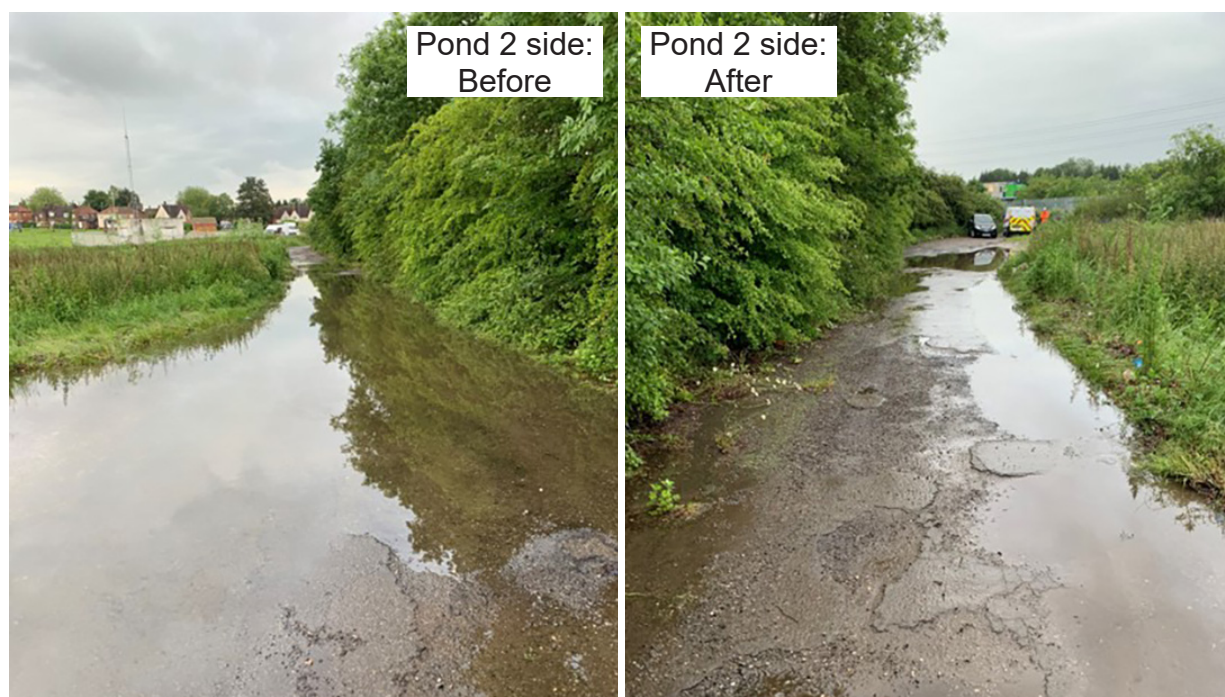
Figure 13: The drop in the water level on the path. Left image shows the path next to pond 2 before blockages were cleared and right image (looking in opposite direction) shows the path after the blockages were cleared (images courtesy of CML).
