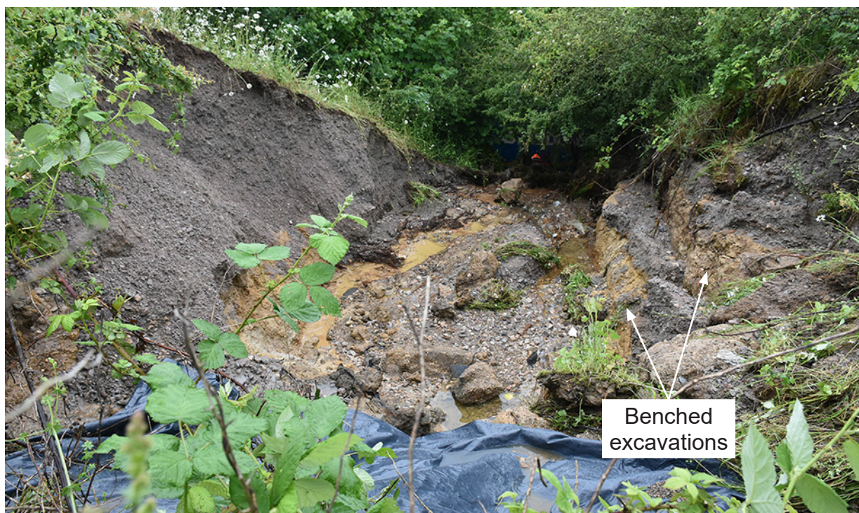
Figure 20: The void left in the cutting slope showing the benched excavations from the 2009 repair, viewed from the top of the cutting slope looking towards the railway
