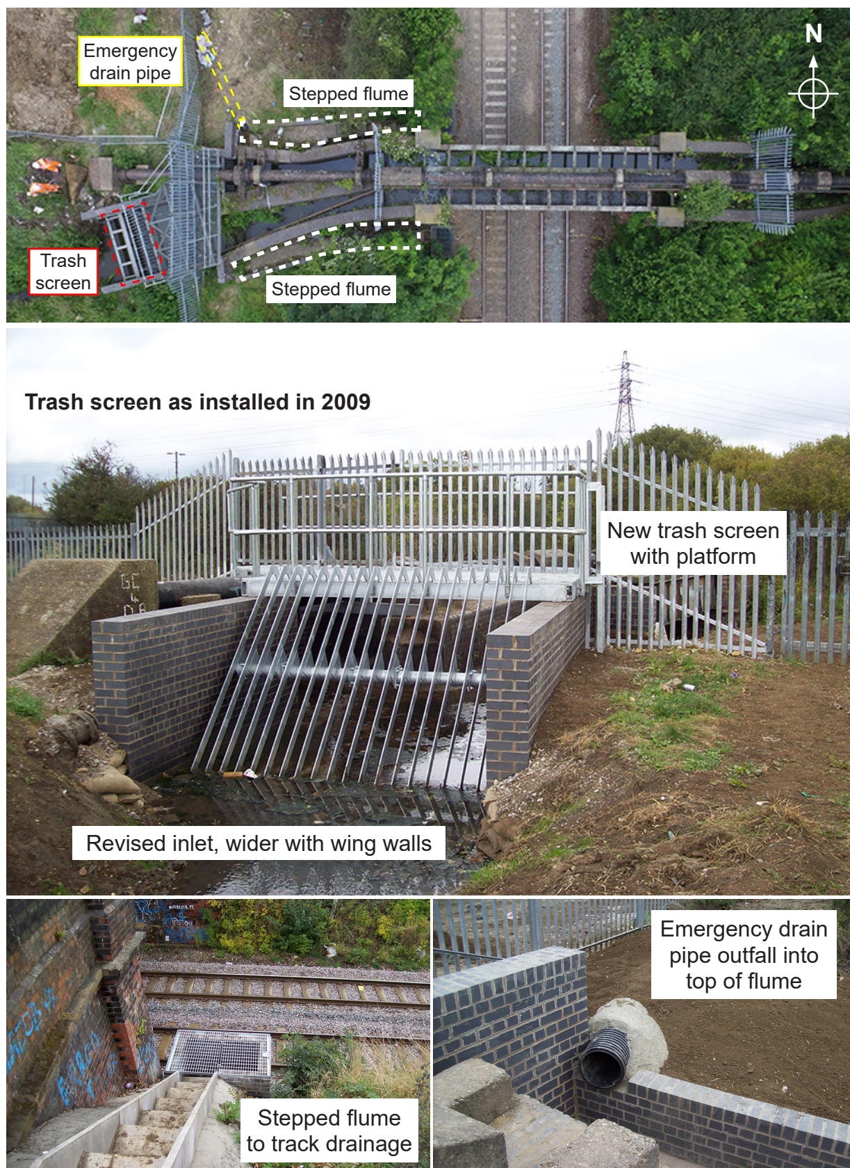
Figure 18: The changes made at the aqueduct's entrance, 2007-2009 (images courtesy of Network Rail)
