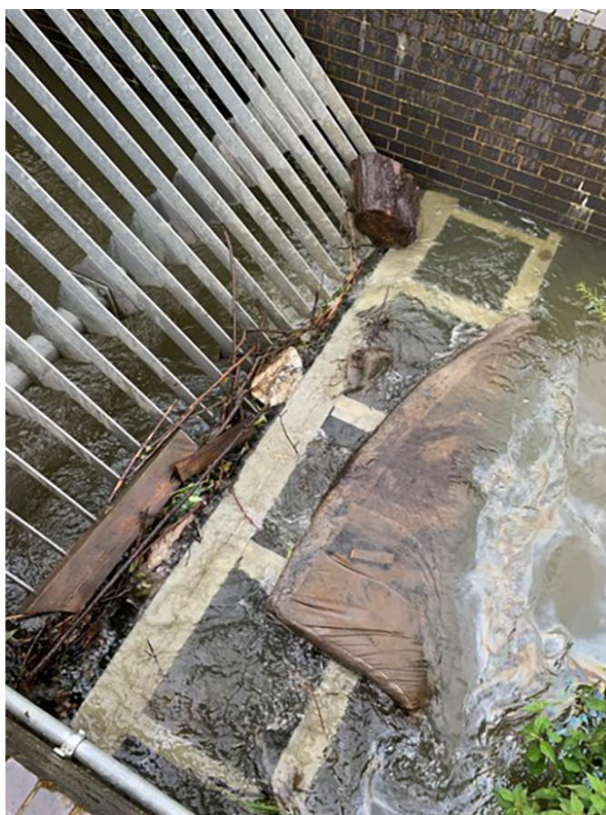
Figure 23: Debris in the aqueduct's trash screen after the incident (image courtesy of CML)
