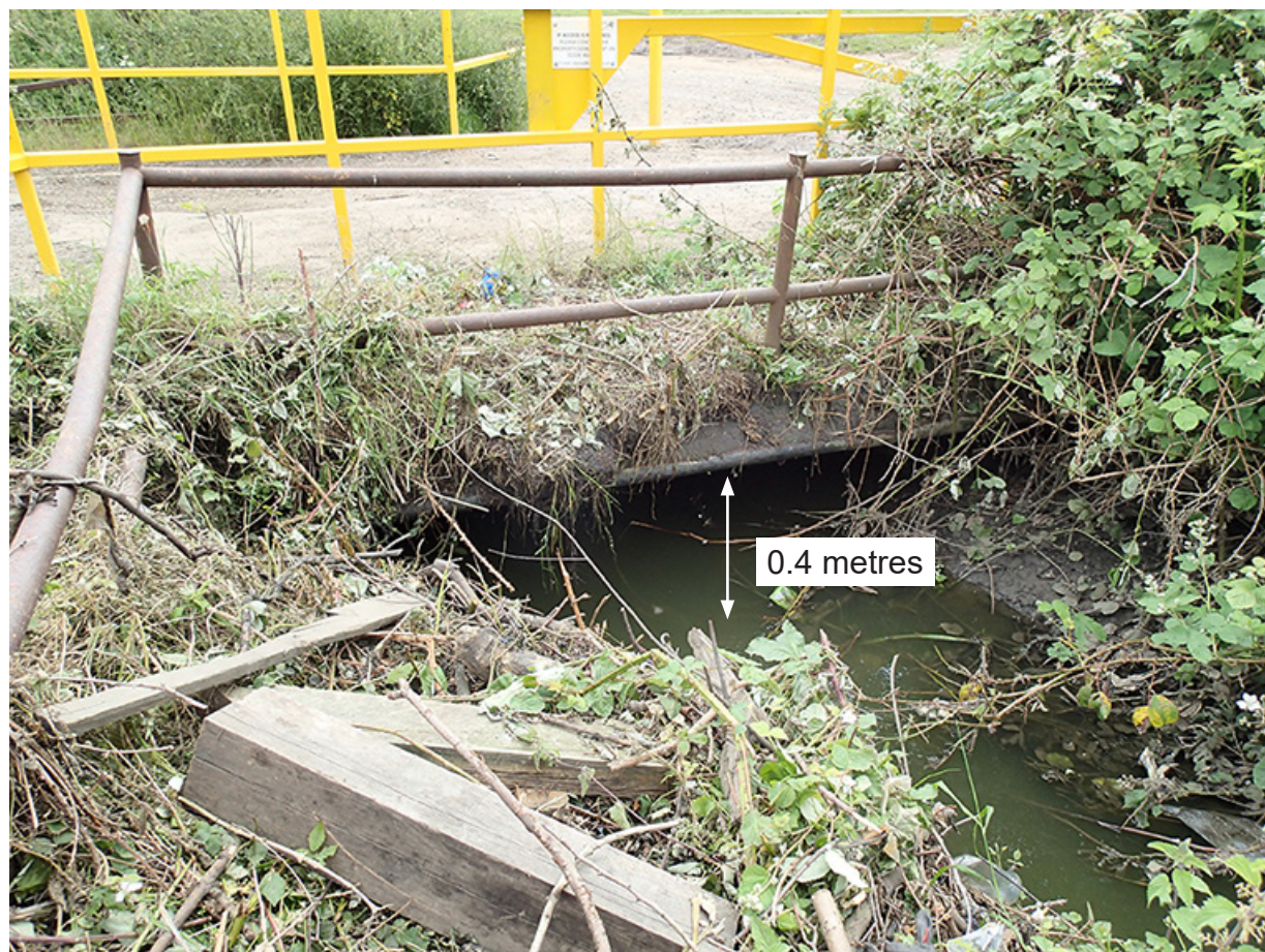
Figure 11: Typical clearance between the underneath of the bridge and the brook when there has been no rainfall for several days
