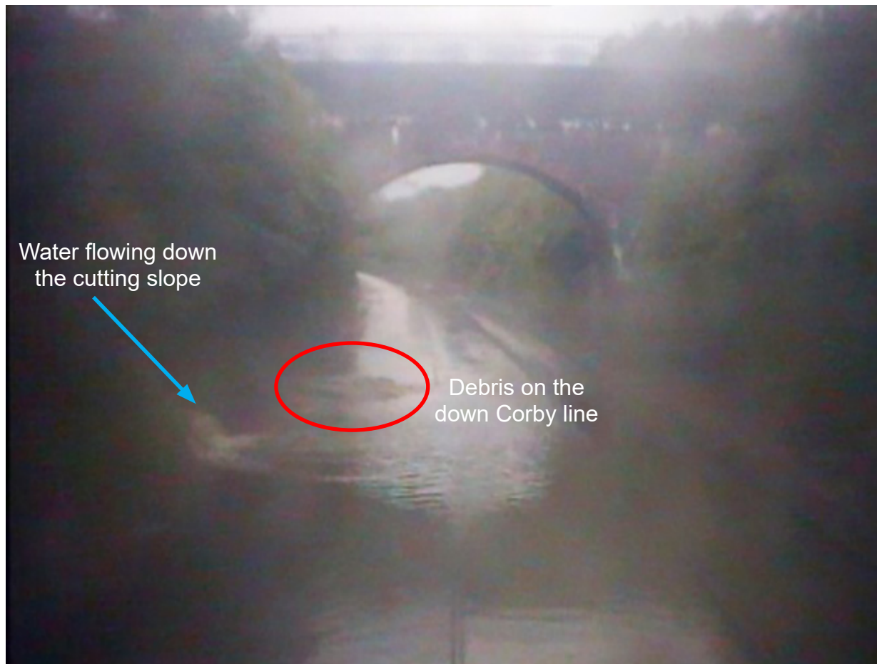
Figure 7: Image from the forward facing CCTV on train 1D43 showing the flooding and debris on the down line.
