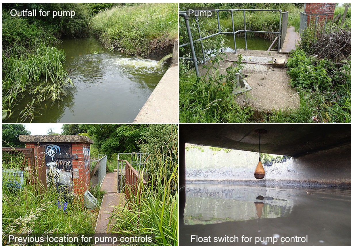
Figure 16: The pumping system at the spillways
