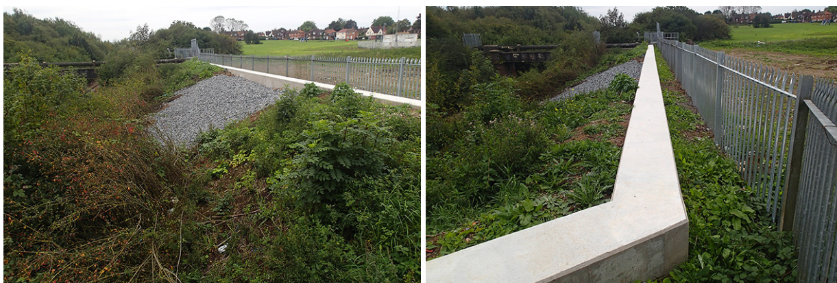
Figure 27: The repaired cutting slope
