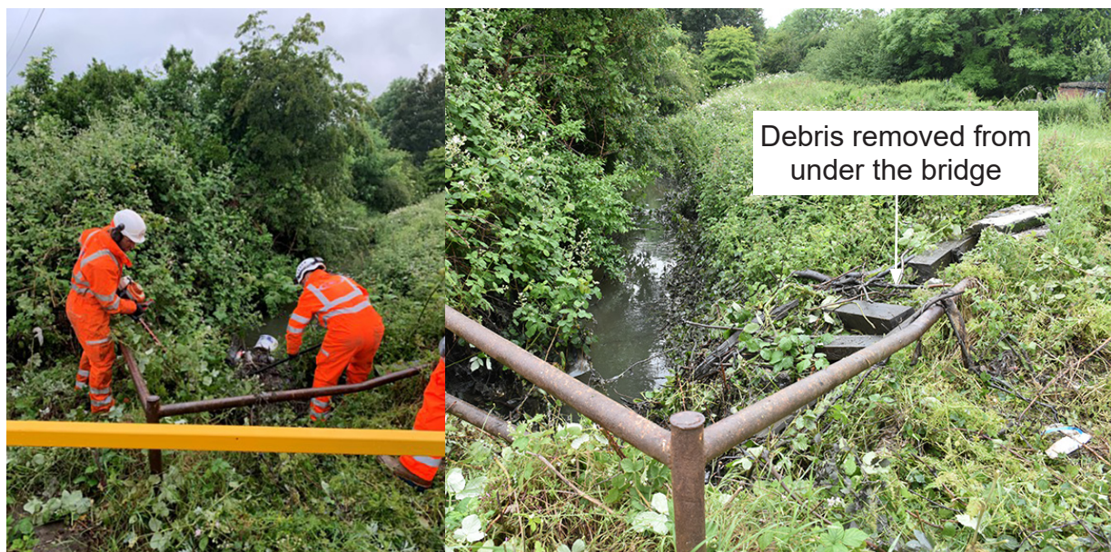
Figure 12: Left image: The contractors called to the site by Network Rail removing debris from the watercourse under and before the bridge (image courtesy of CML). Right image: The debris removed from the watercourse.
