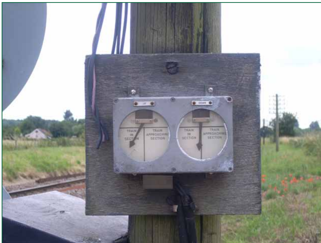
Figure 5: Poplar Farm level crossing indicators (note the up line indicator is showing 'train in section')
