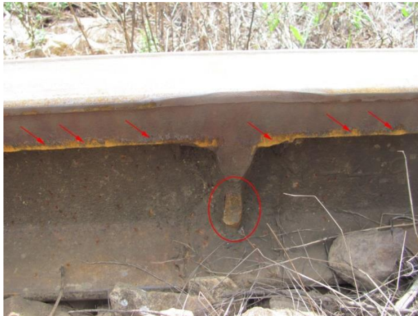
Figure 4.1.6: Traces on the left rail in the direction of motion, at 25 m after the point where the left wheel fell in
