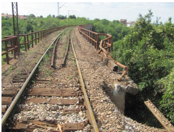
Figure 4.1.9: Point where the wagon hit the beginning of the concrete structure of the bridge
