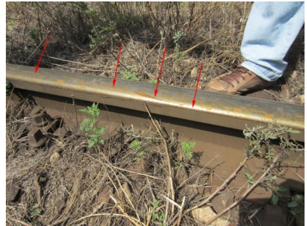
Figure 4.1.7: Traces of the first derailment of the right wheel at 25 m after the point where the left wheel fell into the track
