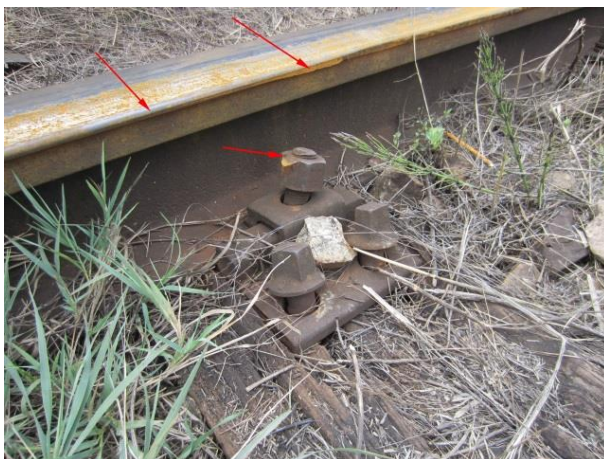
Figure 4.1.4: traces at sleeper 1L
