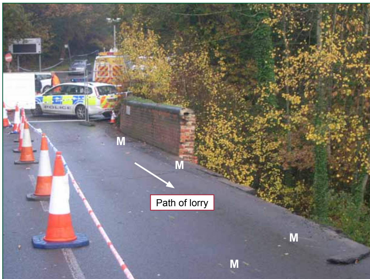
Figure 5: Photograph of bridge deck showing missing section of parapet and skid marks denoted 'M'
