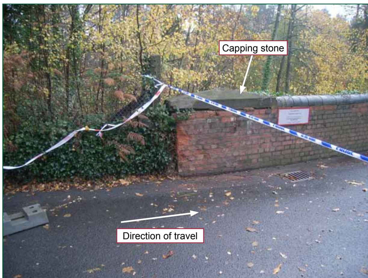
Figure 4: North end of the east parapet which was struck by the lorry
