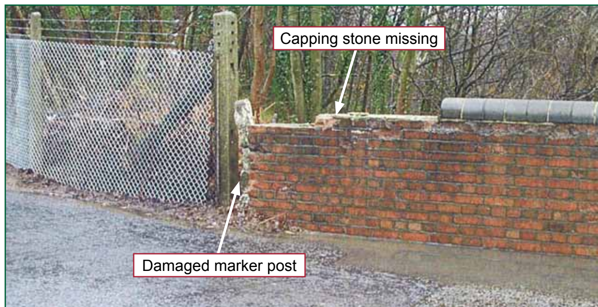
Figure 10: Photograph of the north end of the east parapet showing 'new and longstanding damage' after a similar collision in December 2003 (photograph January 2004, courtesy of Network Rail)
