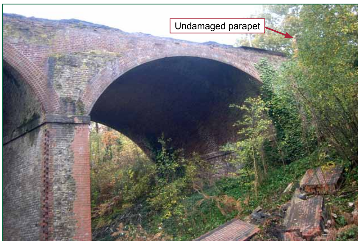
Figure 13: View of bridge and missing parapet from track level. The parapet fell in sections weighing up to 1800 kg
