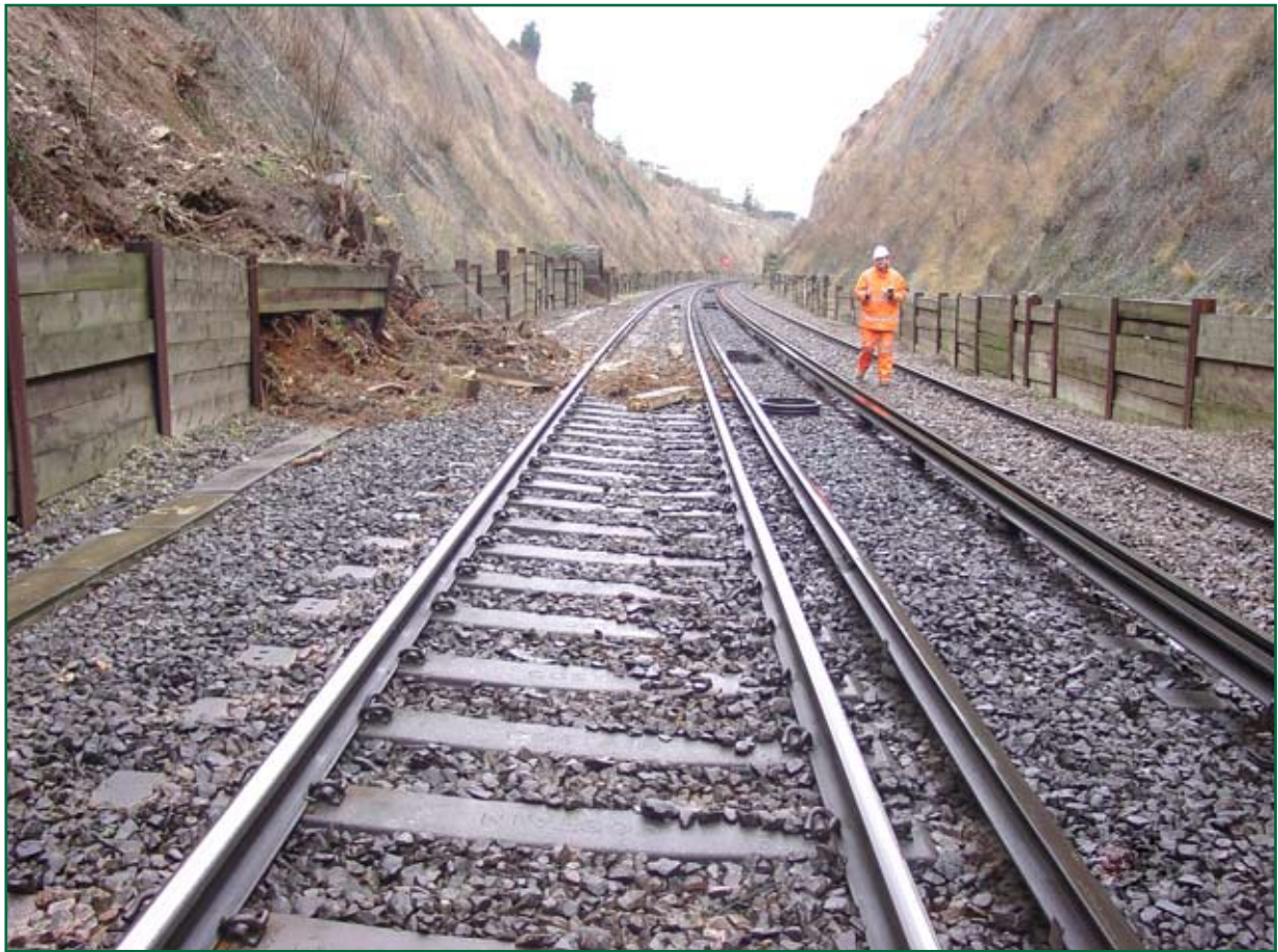
Figure 8: Hooley cutting following the derailment showing the king post wall viewed looking towards London.
