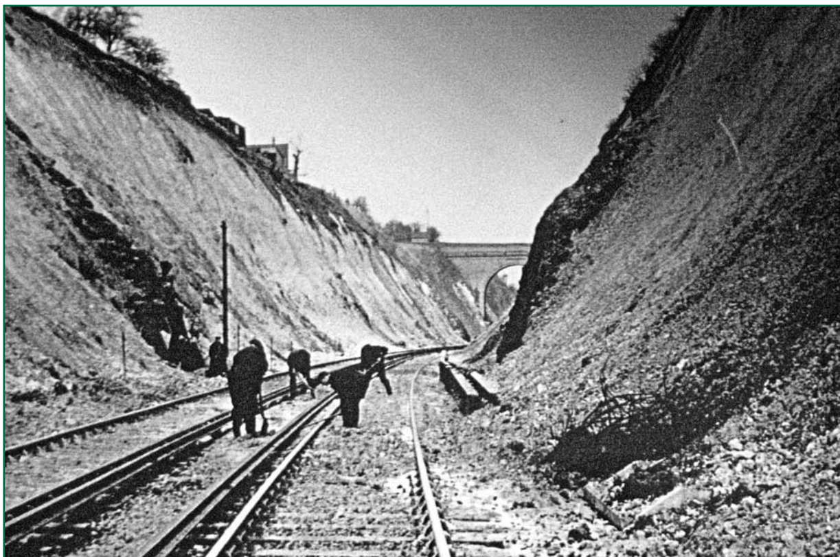
Figure 5: A rock fall on the down side of Hooley cutting during the snows of 1947. The variable depth of gravel can easily be seen on the left side of the cutting (courtesy of Network Rail)
