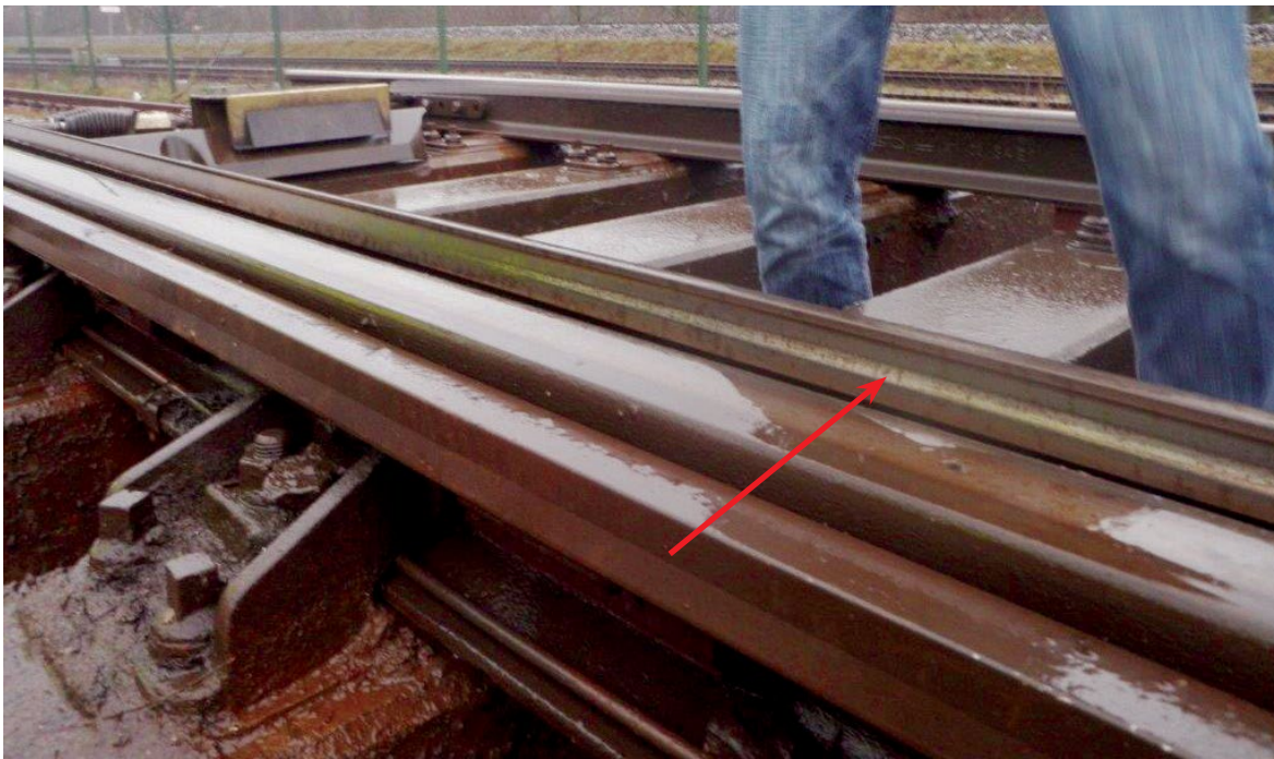
Figure 30: This photograph shows considerable flange-back contact marks on the right-hand switch blade of switch 3B. (Source: ProRail)
