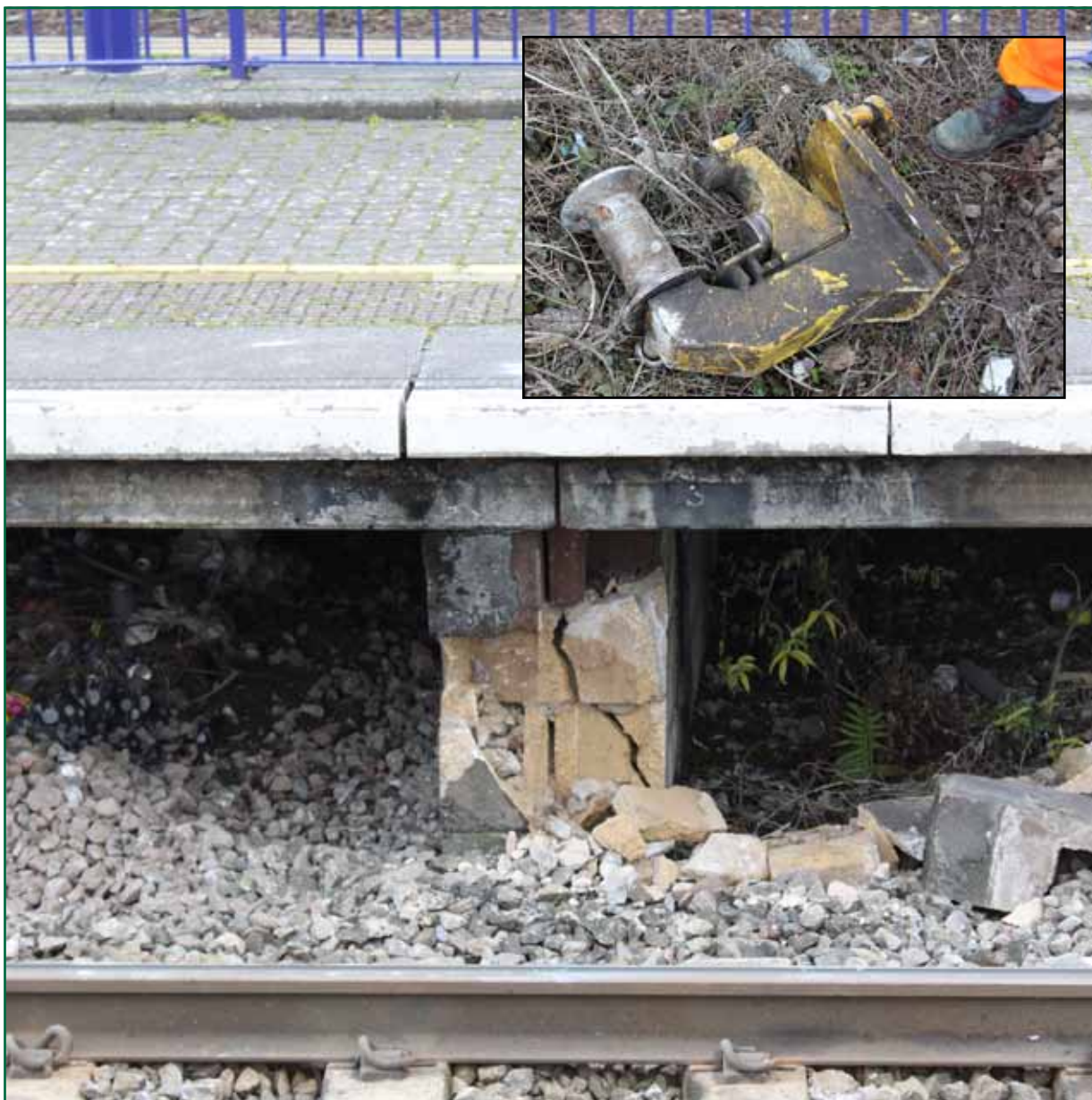
Figure 21: The damaged brick platform support at Thatcham station and the detached clamp (inset)
