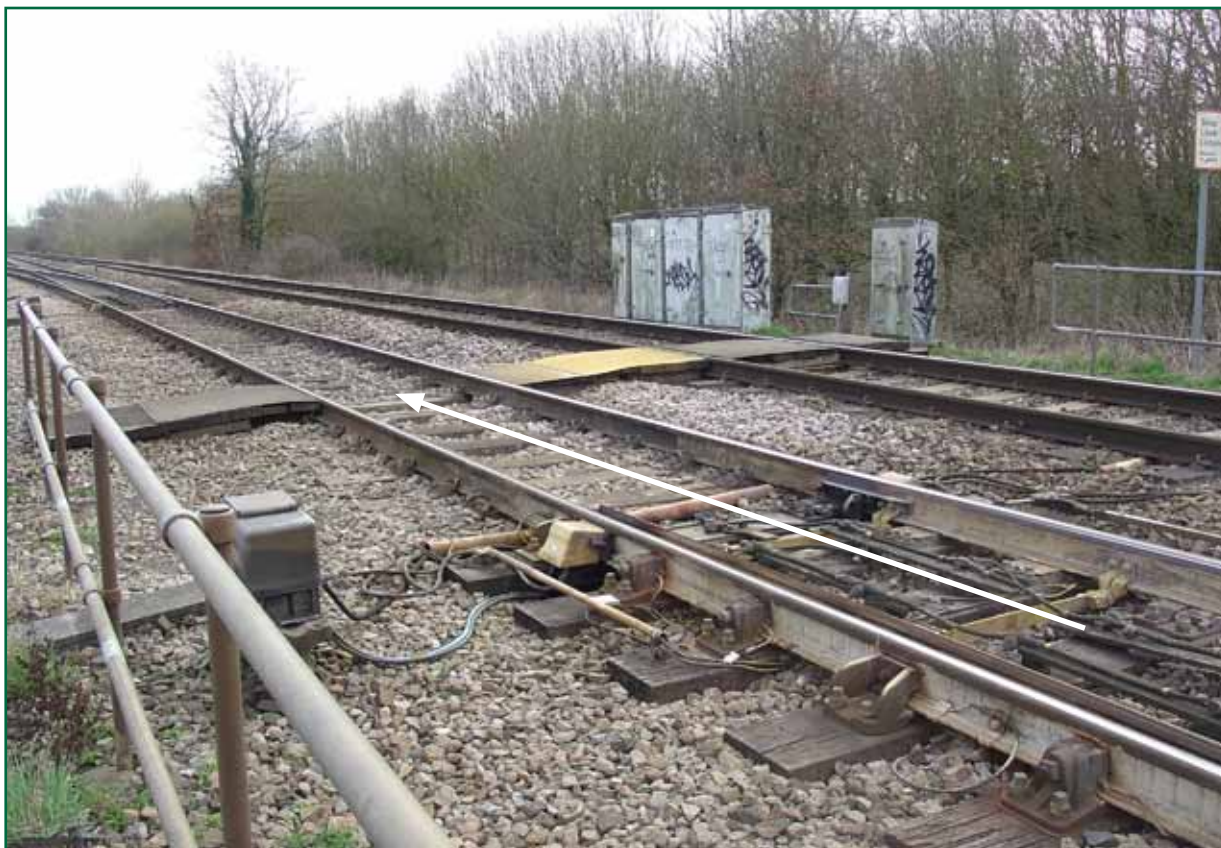
Figure 6: Blatchbridge Junction and the partially destroyed foot crossing (path of train 6Y33 indicated by white arrow)
