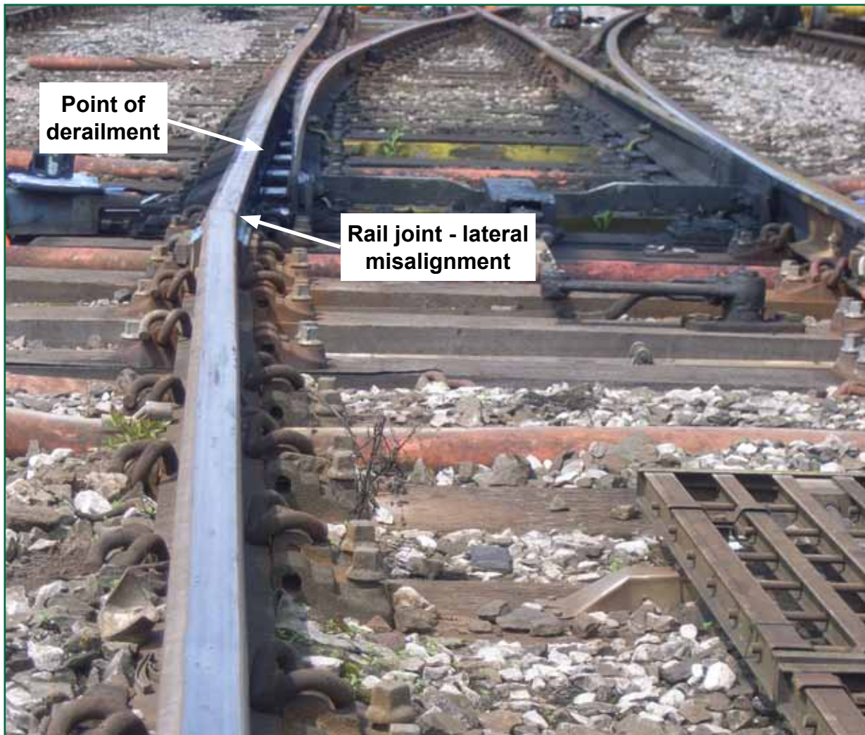
Figure 8: Track lateral alignment approaching No. 75 points
