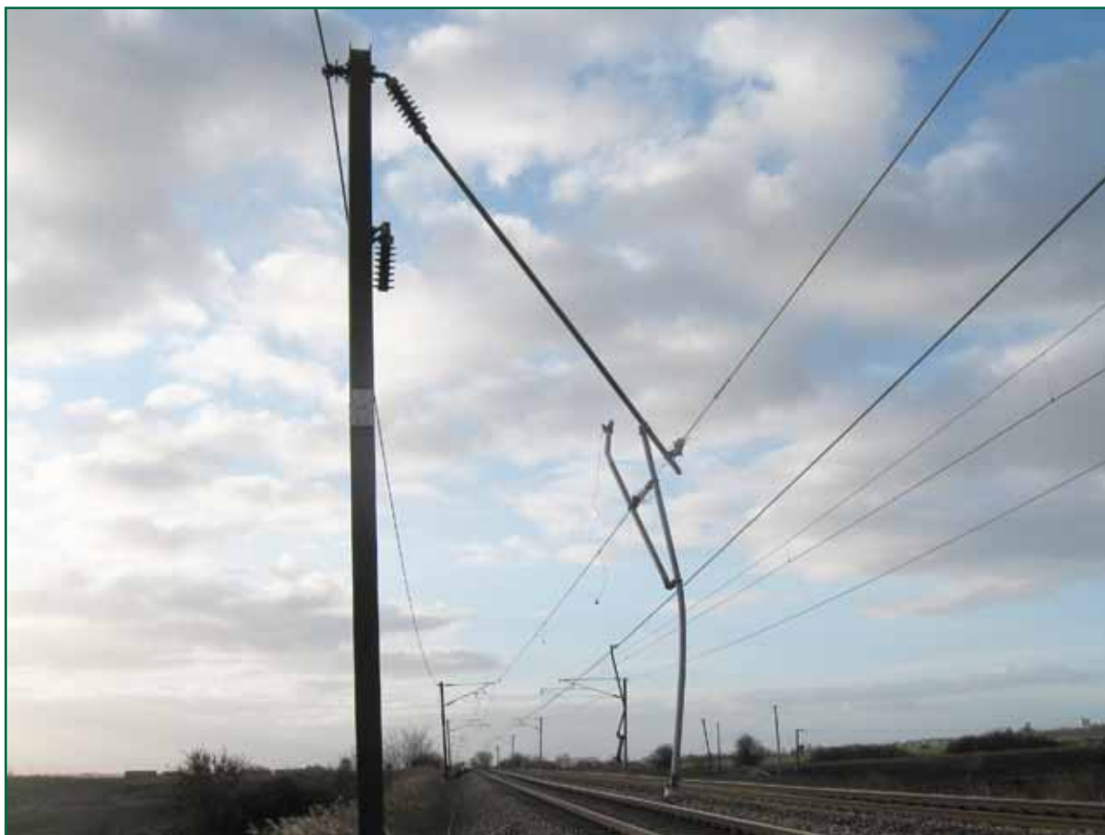
Figure 4: Support structure hit by the pantograph, at mast C118/32 (courtesy of Network Rail)
