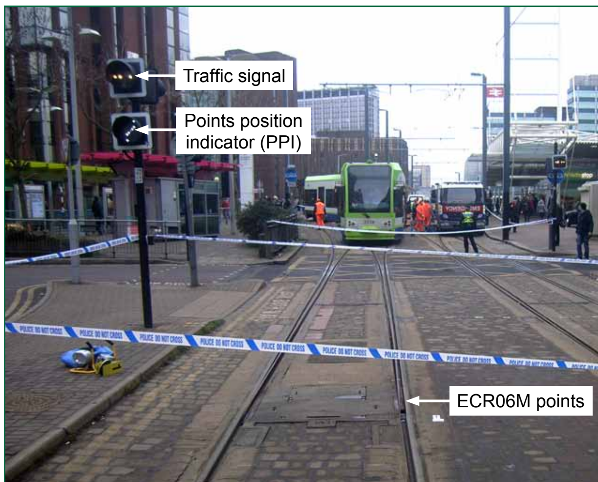
Figure 3: Billinton Hill (Post Office Road) crossing showing points ECR06M, the traffic signal (showing a horizontal row of lights indicating 'stop') and PPI (indicating a route to the right)
