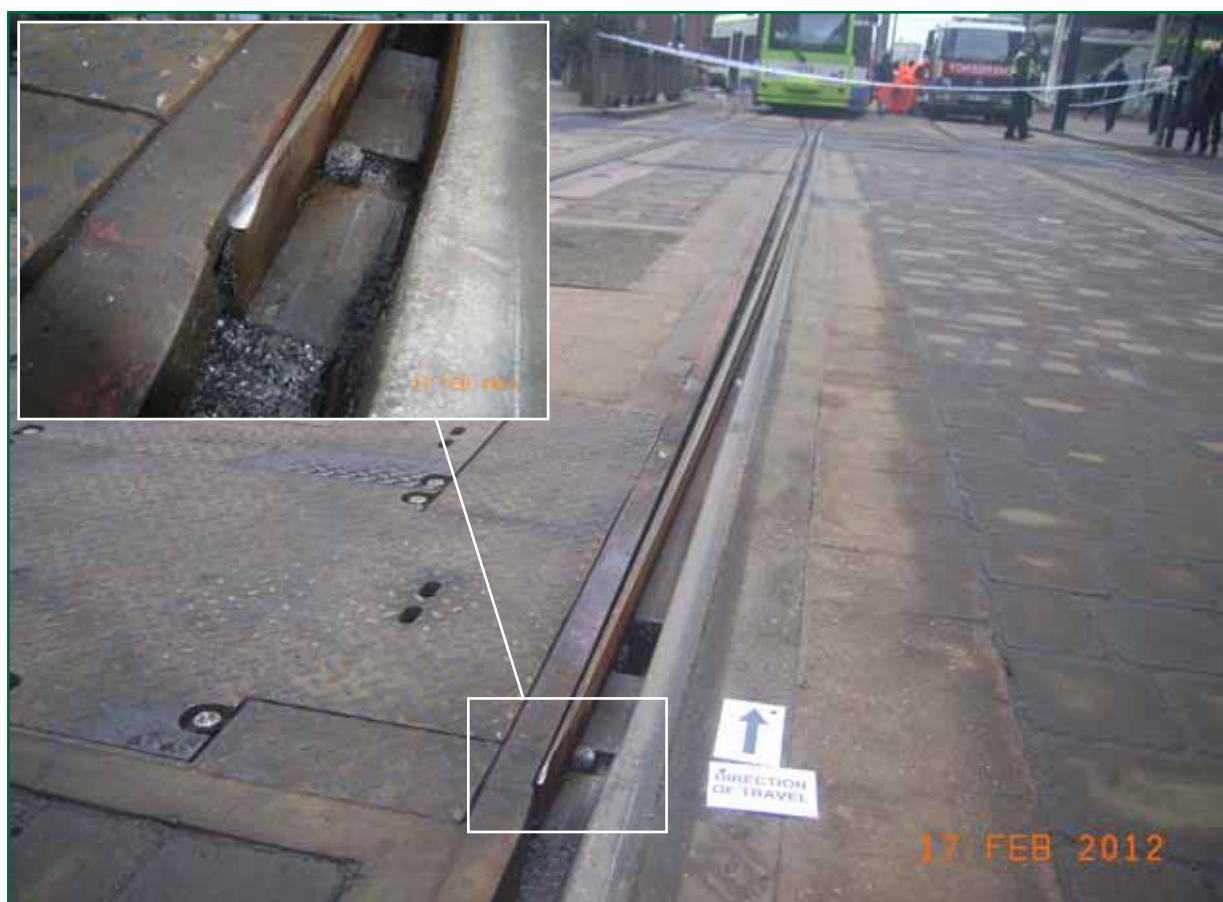
Figure 5: Damage to right-hand switch rail tip (points ECR06M)
