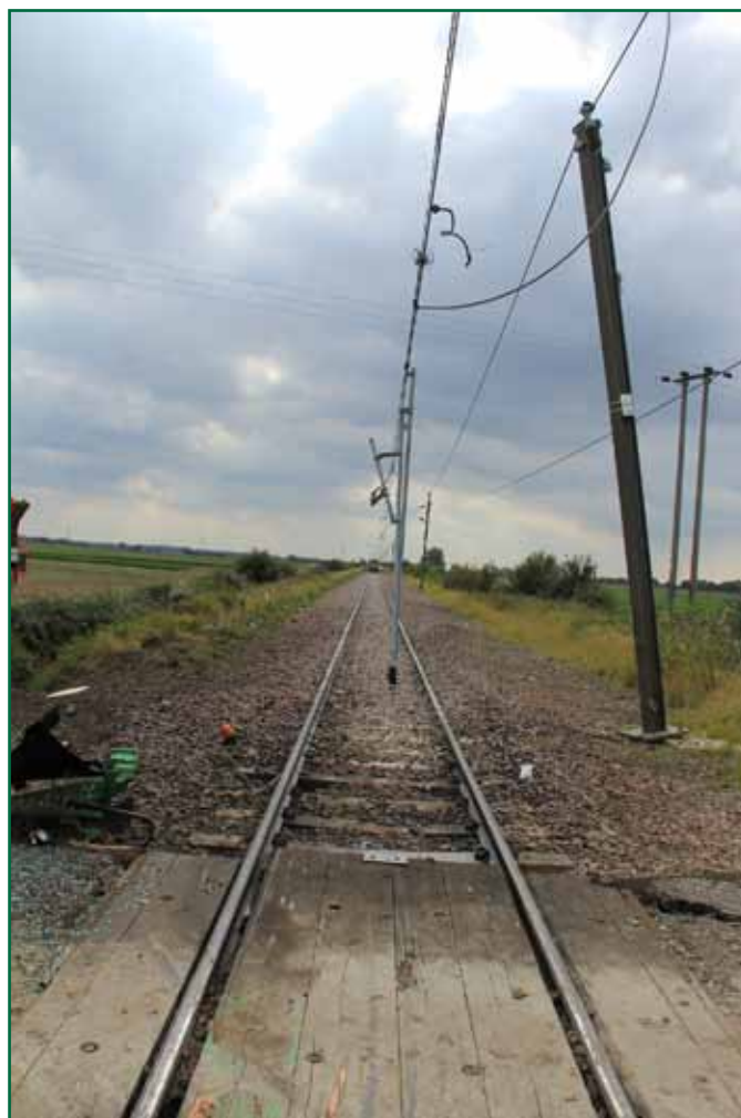
Figure 6: Damage to overhead line stanchion and equipment caused by counterweight from tractor
