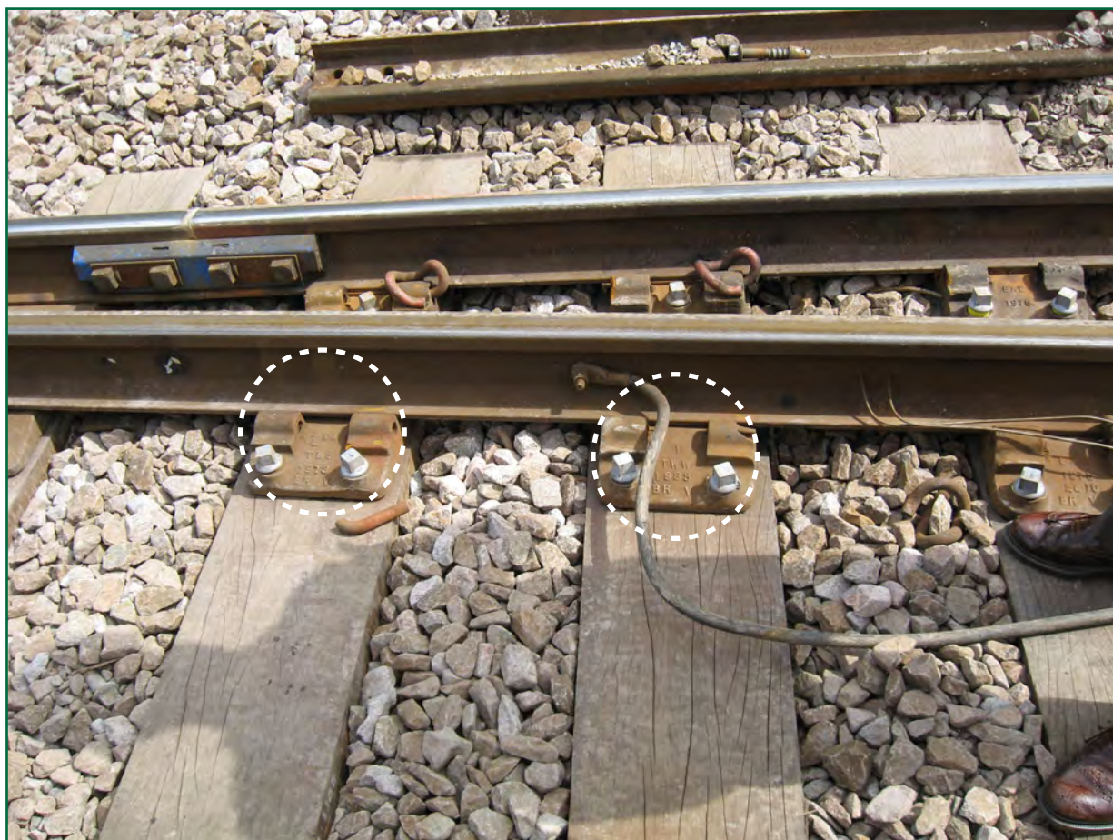
Figure 11: Close up of baseplates with missing fasteners
