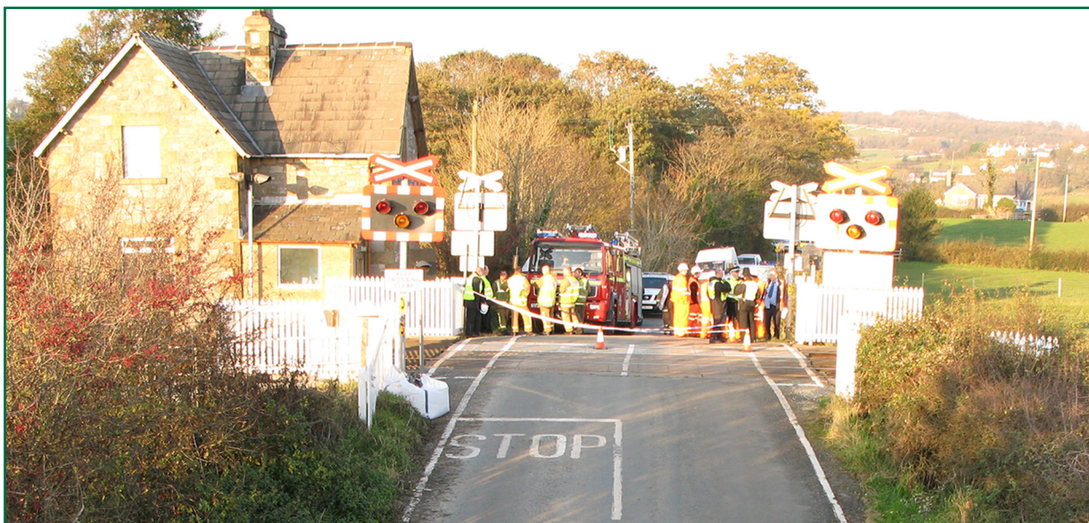
Figure 9: Sunlight reflected off the right-hand signal backboard and warning signs (photograph courtesy of Cumbria Constabulary)
