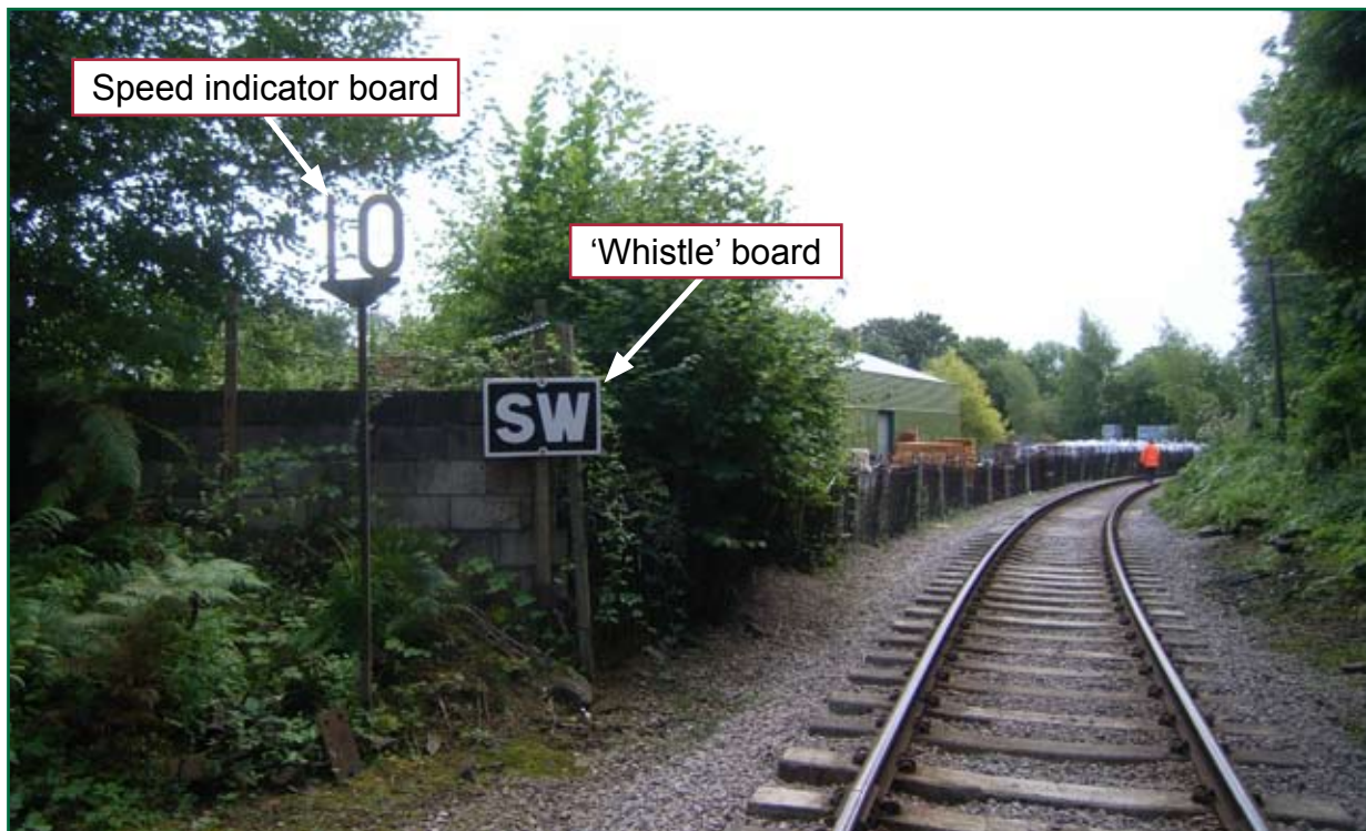
Figure 7: Speed indicator board and 'Whistle' board
