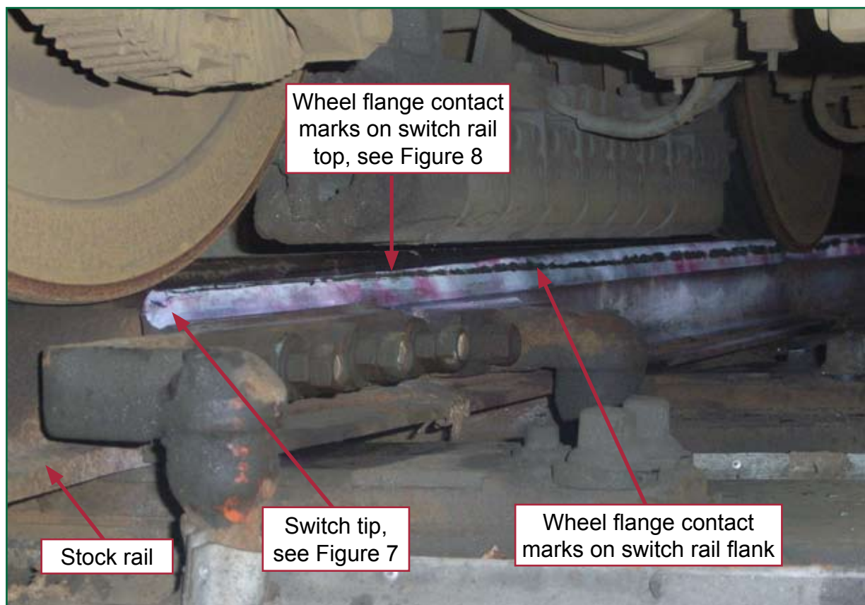
Figure 12: Wheel contact marks in residual dye penetrant material
