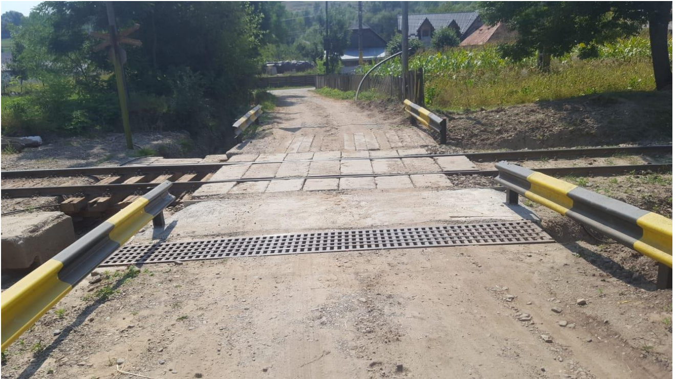
Photo no.3 – level crossing km 4+925, after finishing the rearrangement works
