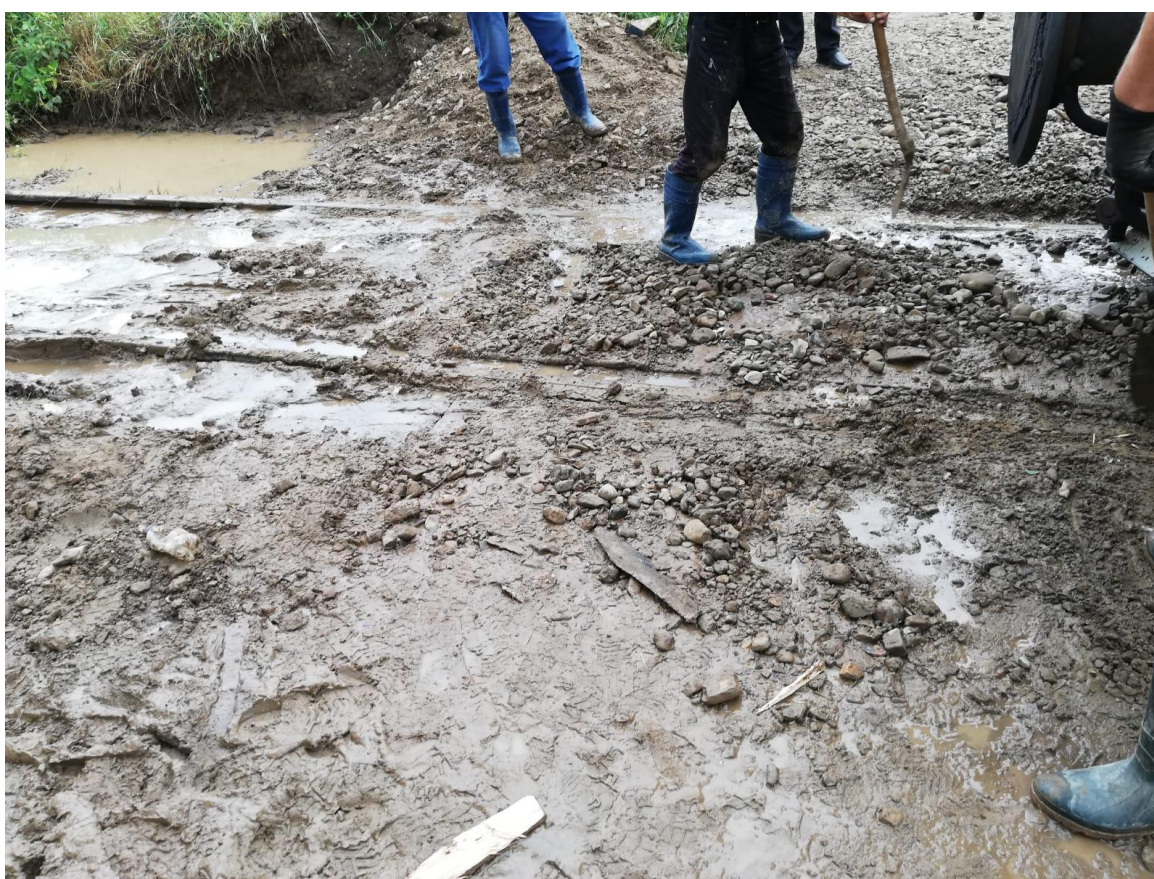
Photo no.1 – removal of the ballast from the level crossing
