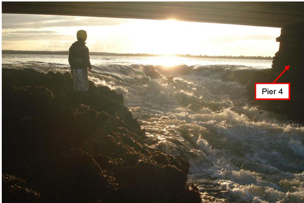
Photograph 9 – Deepened channel between Pier 4 and Pier 5
