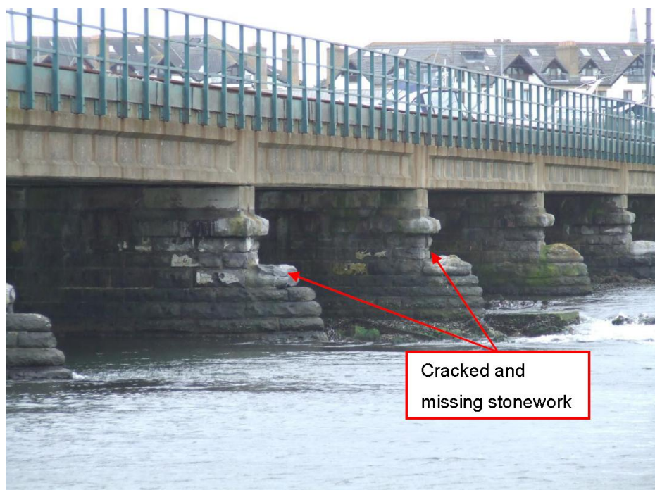
Photograph 15 – Photograph taken by the AE on the 18 th August 2009, showing defects to piers' stonework
