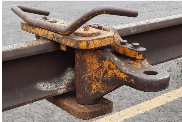
Figure 2 – Clamp fixed to rail
