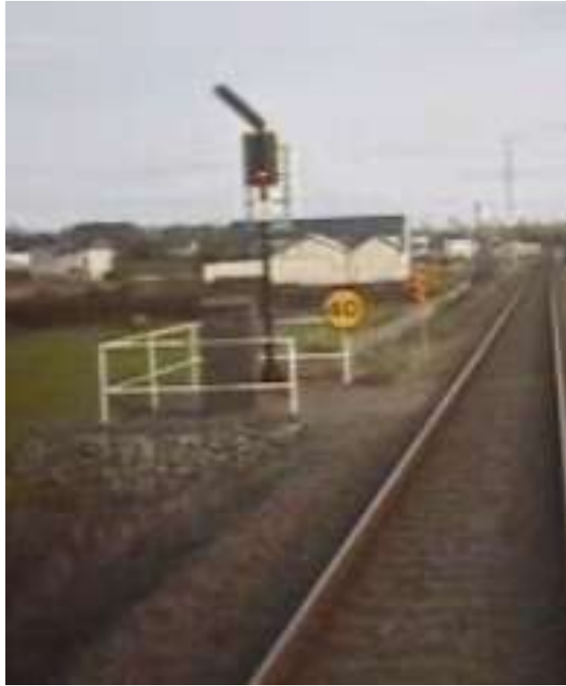
Figure 36 – Signal TL223 & speed board
