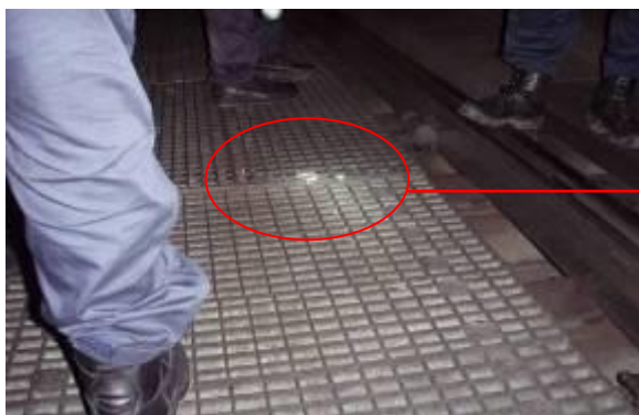
Figure 10 Signs of shear in Blisadona Tunnel
