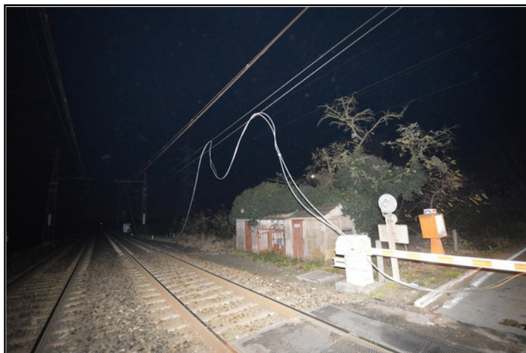
Figure 16 : Feeder arraché
