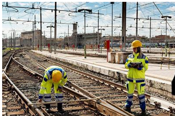
Visual inspections Manual measurements
