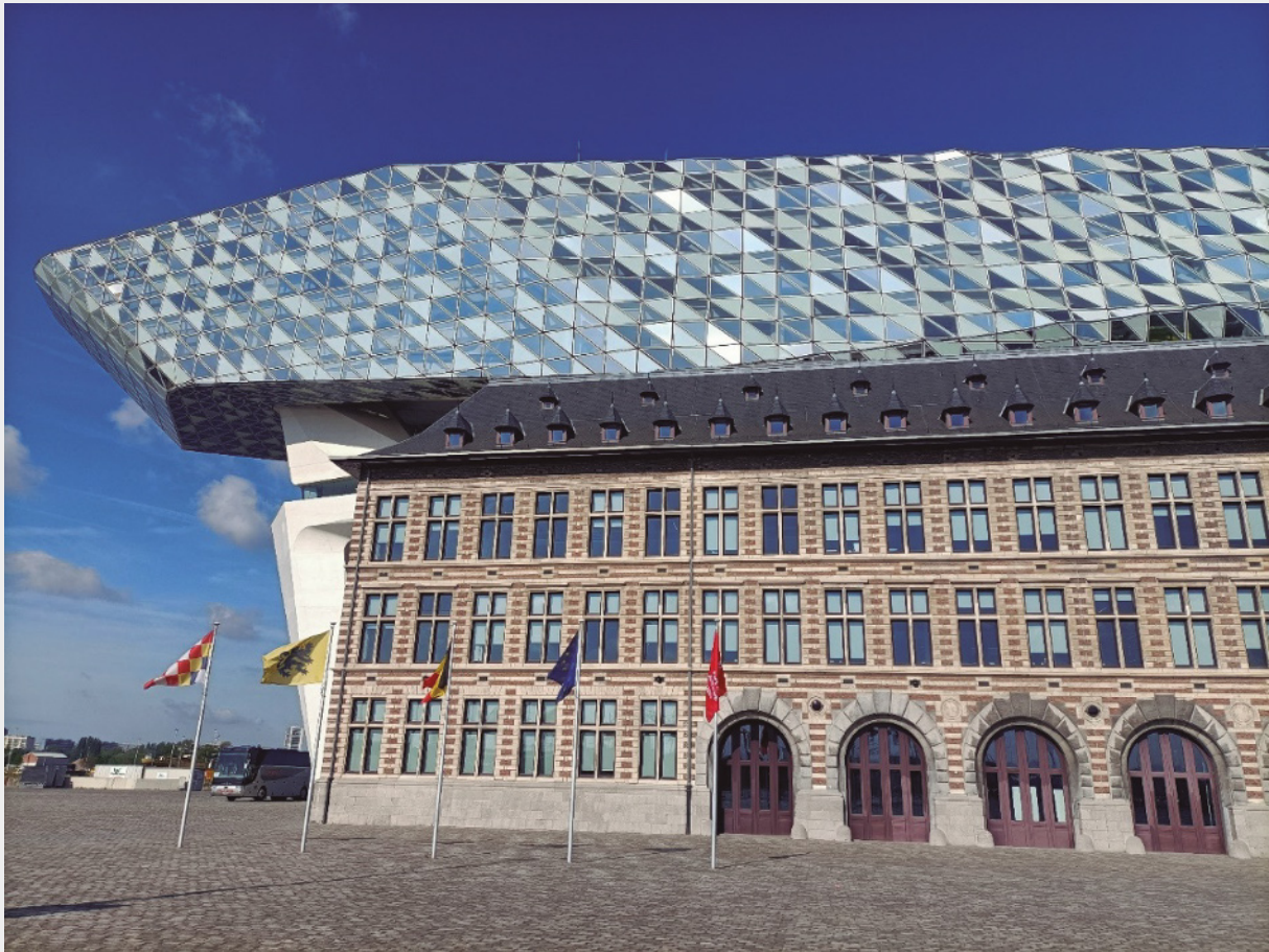
Figure 23: The Havenhuis, the headquarters of the port authority of the Port of Antwerp–Bruges
