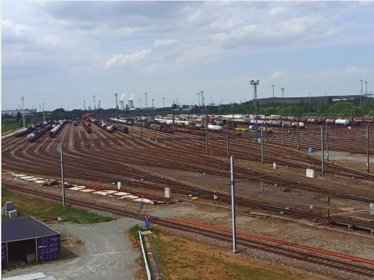
Figure 25: Shunting yard of Antwerp North
