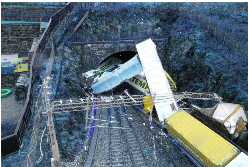
Derailed wagons in the tunnel opening of the Arnanipa tunnel. Photo: NSIA
