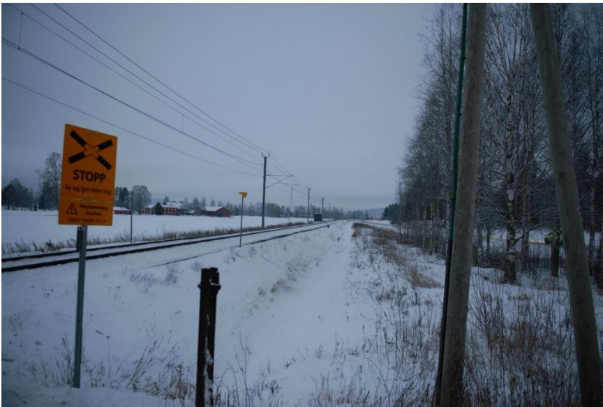
Line of sight from the level crossing in the direction from which the train came. Photo: NSIA
