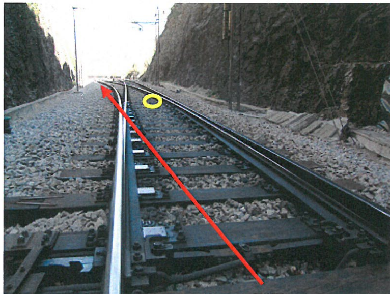
Photo 5: The red arrow shows the travelling direction of train no. 47913 over point no. 1, while the yellow circle shows the break point of the right blade. The blade broke between sleepers 11 and 12.
