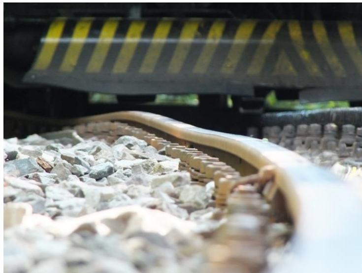
The track distortion at the derailment point
