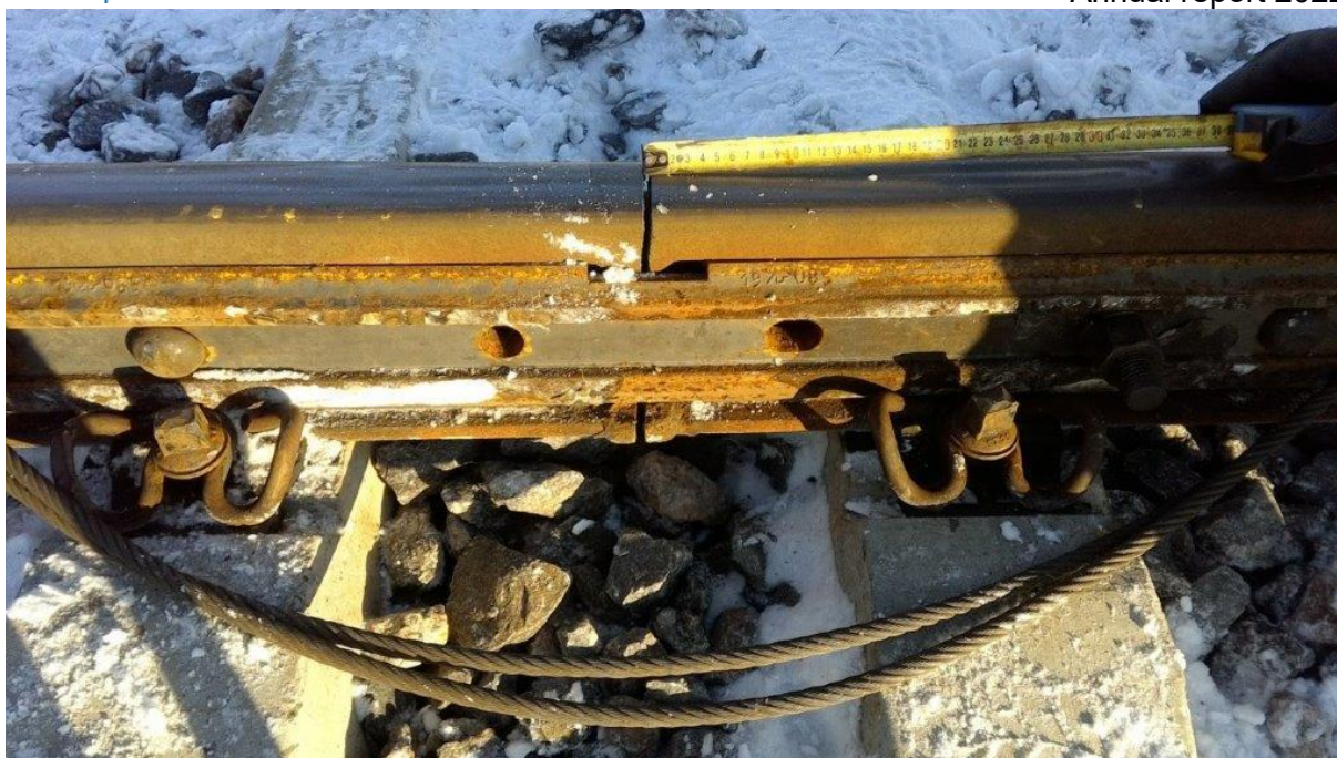
Photo 2. Track breakage in Paldiski 06.12.2021
