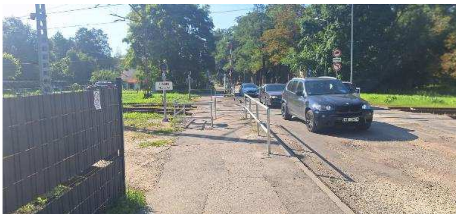
Figure 14. Pedestrian movement control barrier installed after the accident. View from the Akāciju iela side
