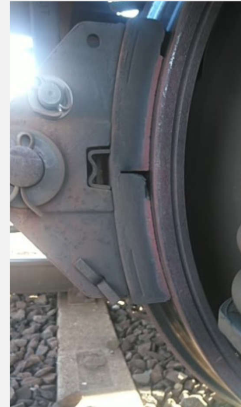
Organic brake blocks: 'Red layer' in the rubbing surface
