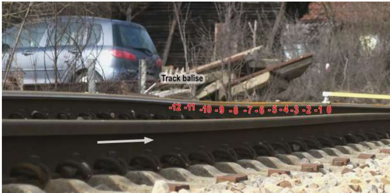
Figure 4.2.8.4: Track layout in the derailment zone
