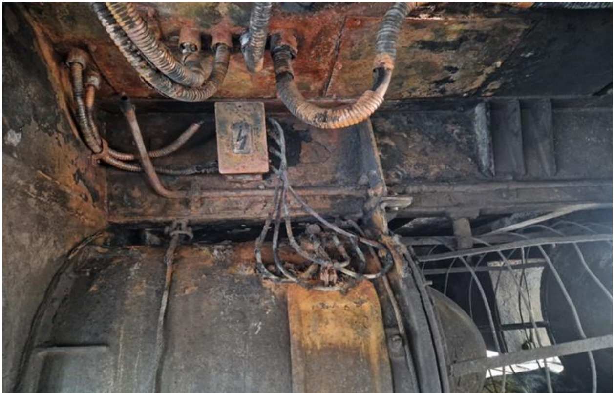
Fig. 4.17. Power supplying cables on the engine-fan, supplied by the terminal box.
