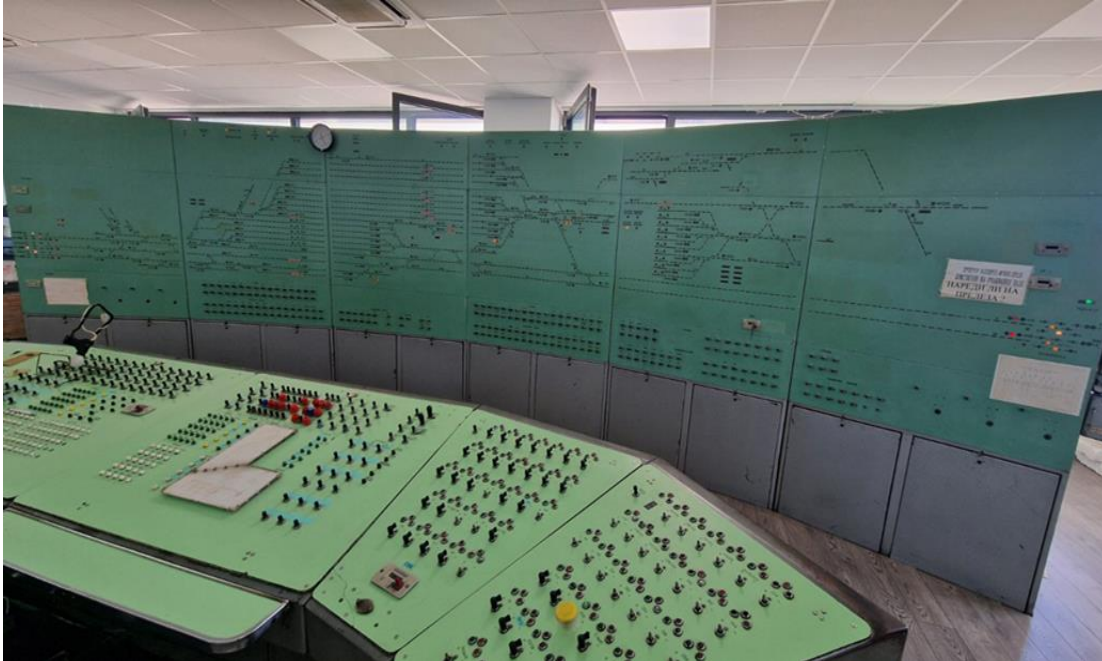
Fig. 3.6. RRI Stara Zagora station with type, Russian block with route shunting“.
